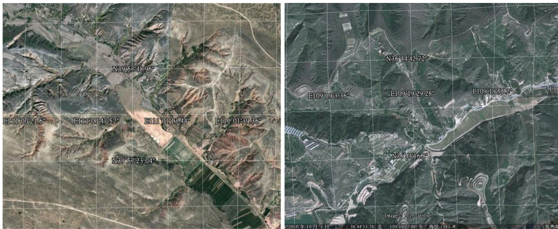
Fig. 2 Check-dam views in the Loess Plateau by Google Earth
